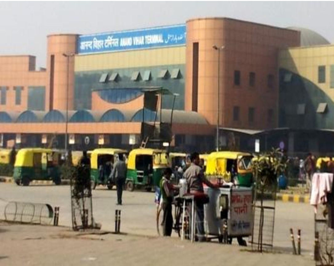
Anand- Vihar: Existing Station Building
